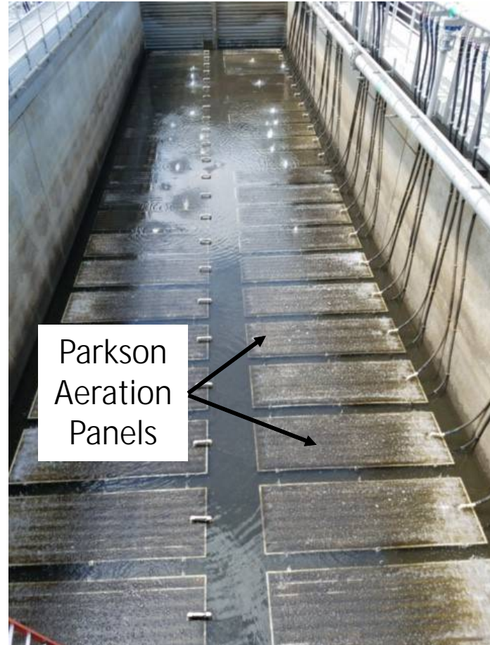
Aeration Basin Out of Service
